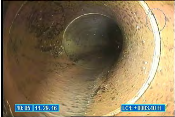
3940_38f2c972-04e0-4cf6-be54-4ea248a8143e.jpg, 00:00:15, 83.40 Tap Factory Made, at 10 o'clock, 6 inch dim
