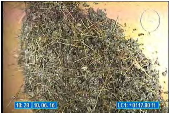
3010_50f36518-9c29-4c5a-ac56-9af001ea76bc.jpg, 00:00:15, 117.80 Roots Medium Joint, from 02 to 04 o'clock, within 8 inch
