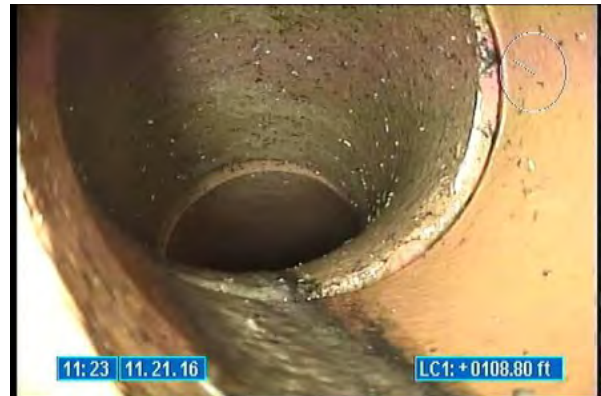
3280_9d340dfd-99d7-4a2d-8cd9-74615205a0df.jpg, 00:00:11, 108.80 Tap Factory Made, at 10 o'clock, 6 inch dim
