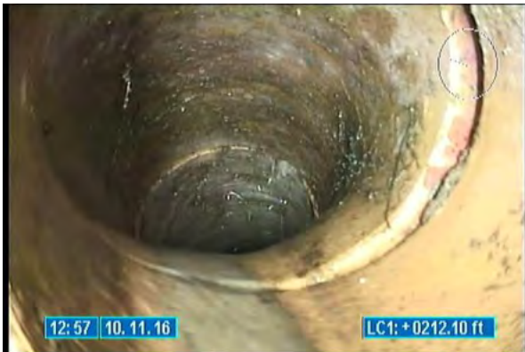
3620_71f74a2f-a395-448b-b642-05be41a52d3c.jpg, 00:00:32, 212.10 Tap Factory Made, at 10 o'clock, 6 inch dim
