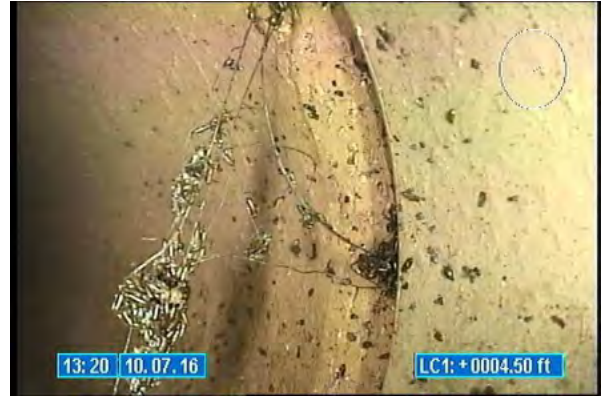
3410_f8181940-dc6c-4612-a128-68d0bbddcfda.jpg, 00:00:02, 4.50 Roots Fine Joint, at 02 o'clock, within 8 inch
