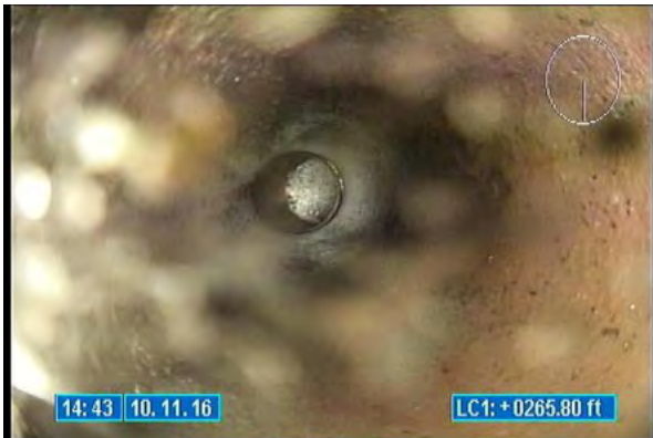
3540_da77d353-846d-47bc-9ca4-cd043addb966.jpg, 00:00:43, 265.80 Tap Factory Made, at 06 o'clock, 6 inch dim
