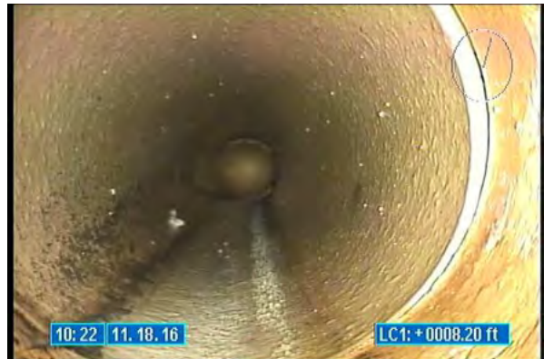
3350_02c3d70a-6b44-44f3-acc8-8422fce7fa43.jpg, 00:00:03, 8.20 Tap Factory Made, at 01 o'clock, 6 inch dim
