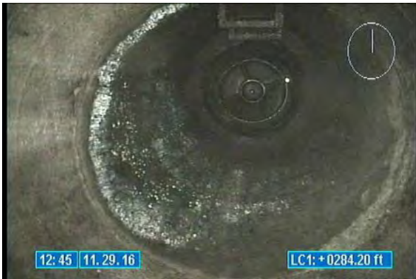
3660_a7cedd30-4b3a-4aa9-8c36-383aa06658c5.jpg, 00:00:23, 284.20 Water Level, Sag in pipe, F01
