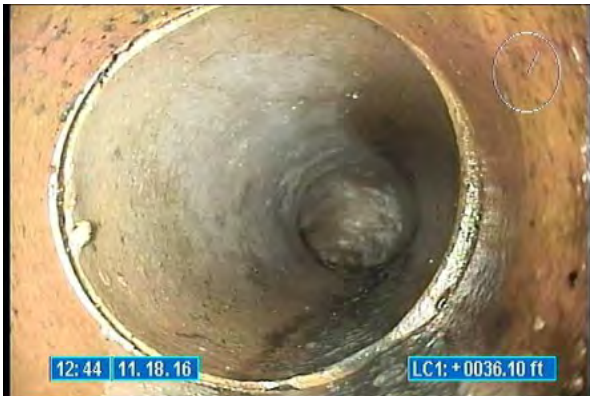
3210_eee3f166-ab83-4c03-9162-f7e3dbdd359a.jpg, 00:00:03, 36.10 Tap Factory Made, at 02 o'clock, 6 inch dim
