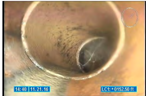
3750_42b8a338-644d-41a5-80df-2313c3f458f6.jpg, 00:00:18, 152.50 Tap Factory Made, at 02 o'clock, 6 inch dim
