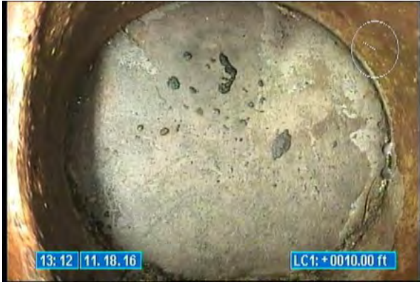
3190_91efedb7-9823-486e-9841-183f1585b48d.jpg, 00:00:01, 10.00 Tap Factory Made Capped, at 10 o'clock, 6 inch dim
