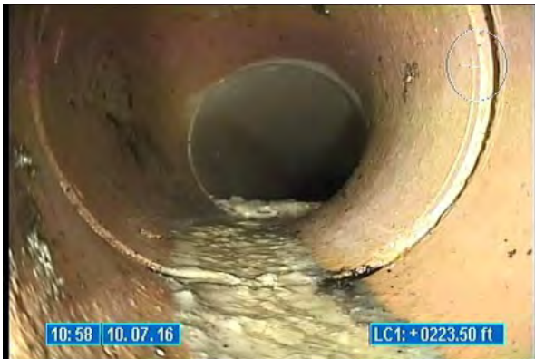
3500_309f7b71-fb42-45f3-b6f3-1a5f92e71eda.jpg, 00:00:32, 223.50 Tap Factory Made Active, at 09 o'clock, 6 inch dim
