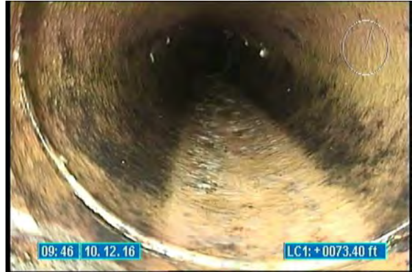
3560_88d48c11-1245-4755-afbe-35e70317584c.jpg, 00:00:46, 73.40 Tap Factory Made Active, at 01 o'clock, 6 inch dim
