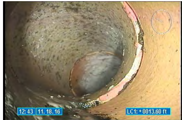
3210_ef02fd62-e4aa-46e7-a4ff-3574319cc6ef.jpg, 00:00:01, 13.60 Tap Factory Made, at 10 o'clock, 6 inch dim
