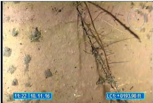
3150_f9af32aa-a18d-4a01-89bb-44ed3bcf4750.jpg, 00:00:21, 193.90 Roots Fine Barrell, at 12 o'clock
