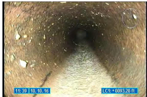
3300_d23f61b9-bb37-4e5f-9542-b22c6c04fcde.jpg, 00:00:20, 93.20 Tap Factory Made, at 12 o'clock, 6 inch dim
