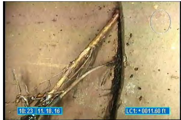
3350_3887208c-2e63-4bc5-9cd1-656ebeeac836.jpg, 00:00:05, 11.60 Roots Fine Joint, at 03 o'clock, within 8 inch
