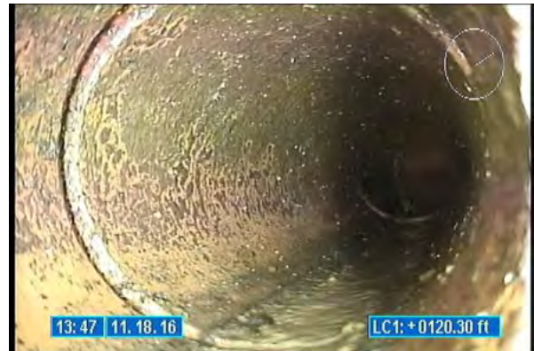
3180_e44d18f7-35e2-4e5c-bfd1-ae4f04e880ca.jpg, 00:00:11, 120.30 Tap Factory Made, at 02 o'clock, 6 inch dim
