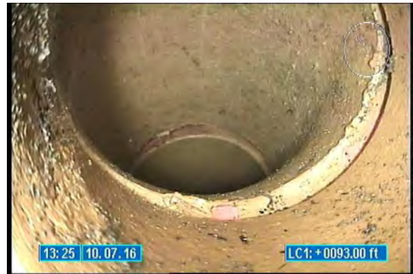
3410_af3ad8e4-07ca-4a33-b5b1-70a0b250d1be.jpg, 00:00:16, 93.00 Tap Factory Made, at 10 o'clock, 6 inch dim
