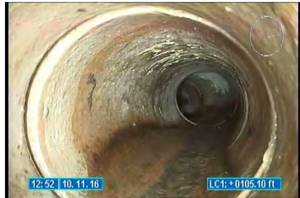
3620_264cf0c7-ddb3-438d-ae1-ee76fd787eab.jpg, 00:00:19, 105.10 Tap Factory Made, at 03 o'clock, 6 inch dim
