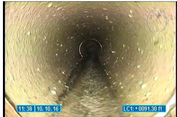
3300_62f7e6ec-0a84-4c66-af20-fba12121a601.jpg, 00:00:18, 91.30 Tap Factory Made Active, at 12 o'clock, 6 inch dim
