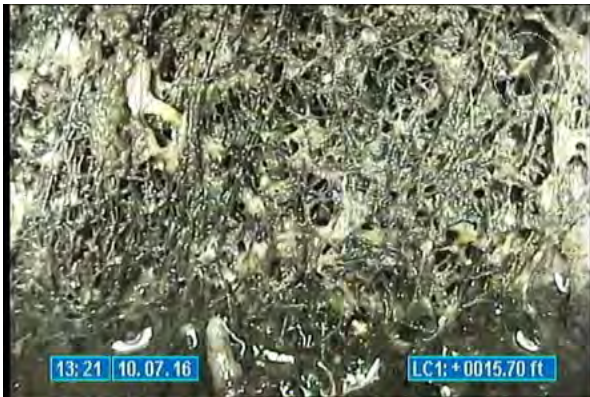
3410_a6a6c1fc-a87e-4026-b5d4-96856385819c.jpg, 00:00:06, 15.70 Roots Medium Lateral, at 03 o'clock
