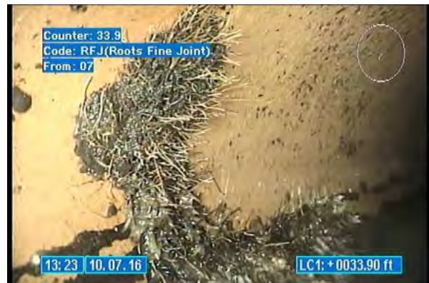
3410_5eabf177-cd50-4f7c-857d-e19d9793fc6b.jpg, 00:00:10, 33.90 Roots Fine Joint, from 07 to 10 o'clock, within 8 inch
