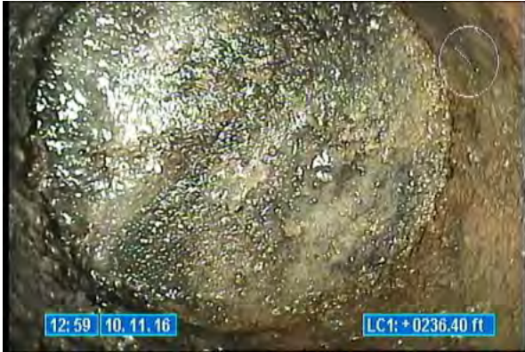
3620_2191137e-35d4-4cdd-830a-d66ac6e3ec5f.jpg, 00:00:38, 236.40 Tap Factory Made Capped, at 10 o'clock, 6 inch dim
