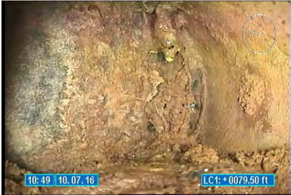
3500_aaf3d719-e6da-40c3-84ec-775dd691524d.jpg, 00:00:11, 79.50 Deposits Attached Encrustation, at 10 o'clock
