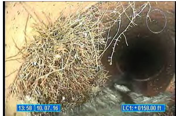
3230_db1121ef-8c97-4286-b28b-4bcac16af369.jpg, 00:00:16, 158.00 Roots Medium Joint, from 07 to 05 o'clock, within 8 inch
