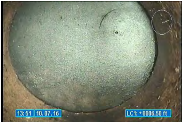
3230_49ee1782-df18-4ac0-a46f-f8e458f3380a.jpg, 00:00:00, 6.50 Tap Factory Made Capped, at 02 o'clock, 6 inch dim
