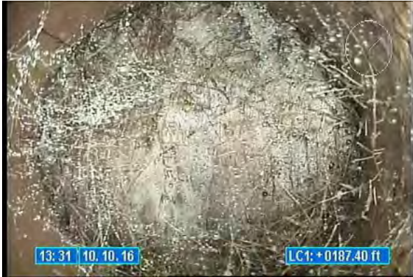
3310_05b0bd53-914d-4f51-97b1-1dd4f6d1ec67.jpg, 00:00:28, 187.40 Tap Factory Made Capped, at 02 o'clock, 6 inch dim
