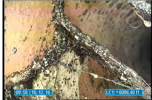
3560_402a3c67-9191-4976-ade3-dde1a2baf16a.jpg, 00:00:56, 96.40 Roots Fine Barrell, from 07 to 05 o'clock
