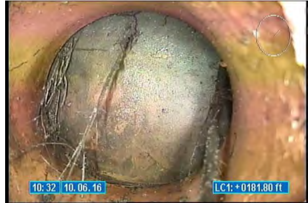
3010_c9272ac5-5b67-4d90-9f01-f911c336ca44.jpg, 00:00:23, 181.80 Tap Factory Made Capped, at 02 o'clock, 6 inch dim
