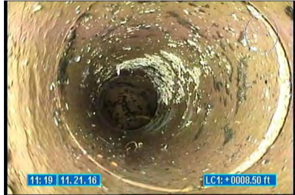
3280_aaa468d1-f3e5-4dd1-9862-1ae95a642f6d.jpg, 00:00:01, 8.50 Tap Factory Made, at 10 o'clock, 6 inch dim
