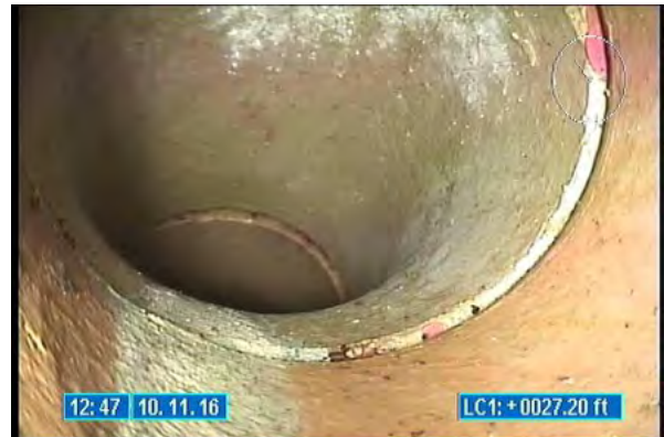
3620_5a03ee69-3e87-403e-8818-d71d297232b2.jpg, 00:00:08, 27.20 Tap Factory Made, at 10 o'clock, 6 inch dim
