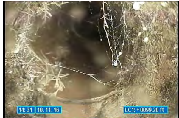
3540_0cef4280-299c-4ae2-9599-0d4a1ba2eb1c.jpg, 00:00:15, 99.20 Tap Factory Made, at 03 o'clock, 6 inch dim
