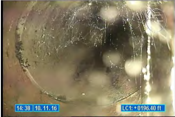
3540_a5463d70-424c-46e9-ab2c-1fd0dfe5a537.jpg, 00:00:31, 196.40 Tap Factory Made, at 03 o'clock, 6 inch dim
