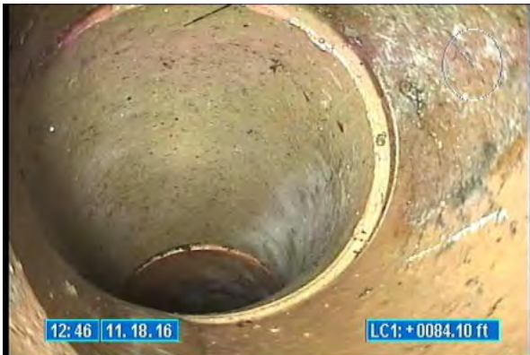
3210_fa6a3951-7180-401b-b9c0-be1fb1ff3bb8.jpg, 00:00:07, 84.10 Tap Factory Made, at 10 o'clock, 6 inch dim
