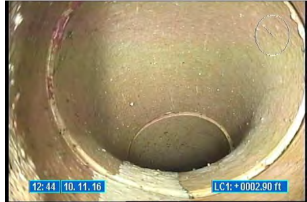
3620_751062fd-33a3-4d21-9e38-2cb380e3ee50.jpg, 00:00:01, 2.90 Tap Factory Made, at 10 o'clock, 6 inch dim
