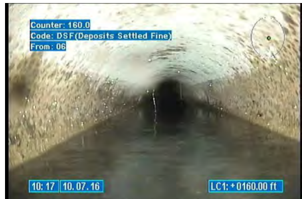
3520_a79bd56c-ac86-4c71-9806-a2334418946c.jpg, 00:00:31, 160.00 Deposits Settled Fine, at 06 o'clock
