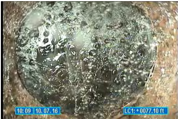
3520_56aa8790-a467-448f-a749-25c291fbed93.jpg, 00:00:15, 77.10 Tap Factory Made Capped, at 10 o'clock, 6 inch dim
