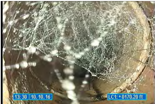
3310_873f5951-527d-4c6d-bd14-a8efd62218be.jpg, 00:00:25, 170.20 Tap Factory Made, at 09 o'clock, 6 inch dim
