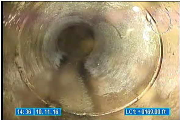
3540_dba867dc-5236-4729-ad27-2697d8c680ed.jpg, 00:00:26, 169.00 Tap Factory Made, at 10 o'clock, 6 inch dim
