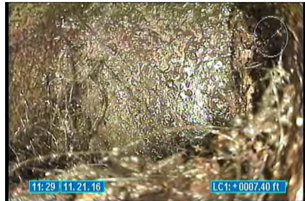
3290_91e65760-4da5-417e-b8e8-3b9390280dff.jpg, 00:00:03, 7.40 Tap Factory Made Capped, at 02 o'clock, 6 inch dim
