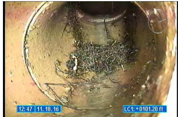
3210_658efefa-f4f2-45fc-b452-26c2a60528f5.jpg, 00:00:09, 101.20 Tap Factory Made, at 03 o'clock, 6 inch dim
