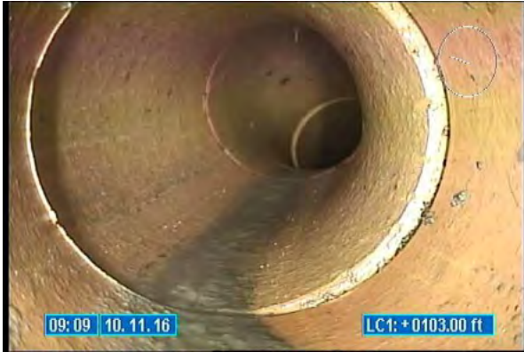
3100_684e3001-691f-4785-93d0-4102ed4fc4cf.jpg, 00:00:14, 103.00 Tap Factory Made, at 10 o'clock, 6 inch dim
