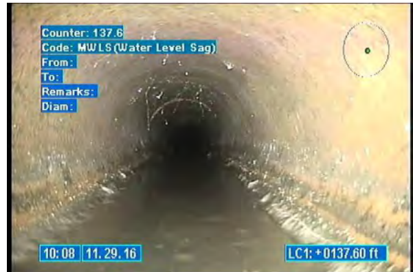
3940_16c99795-1313-47f9-b81d-b294a03a2fa4.jpg, 00:00:22, 137.60 Deposits Settled Gravel, at 06 o'clock
