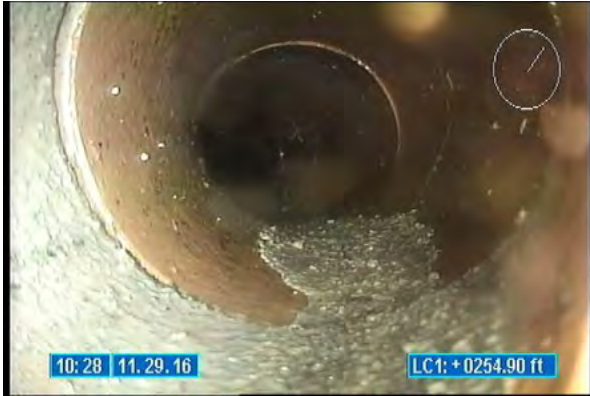
3940_187c7b58-8ea1-4f96-8389-48f85658e08c.jpg, 00:00:55, 254.90 Tap Factory Made, at 02 o'clock, 6 inch dim
