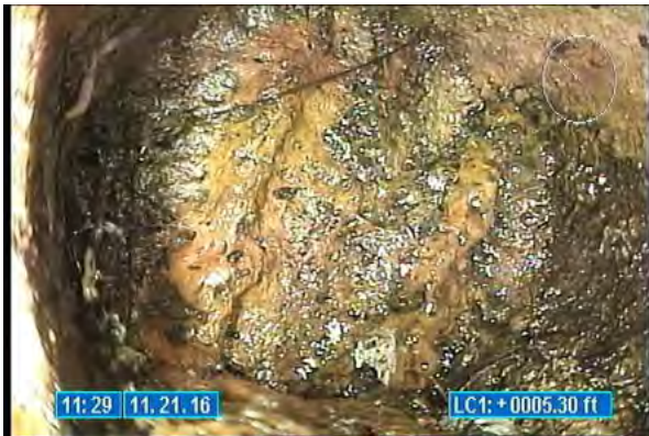
3290_26d783c9-6051-4091-8d43-0c75f35e66c8.jpg, 00:00:01, 5.30 Tap Factory Made Capped, at 10 o'clock, 6 inch dim
