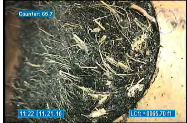
3280_4bb46c9b-f3e0-4514-9a9e-fce6eb829d9b.jpg, 00:00:08, 65.70 Tap Factory Made Defective, at 02 o'clock, 6 inch dim
