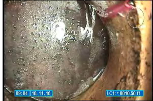
3100_78877973-cdc6-42a0-bffa-56d600a3be76.jpg, 00:00:03, 10.50 Infiltration Runner, at 03 o'clock
