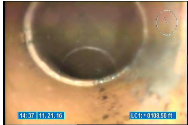
3750_5219058b-ba55-4650-a344-16df8ab27186.jpg, 00:00:13, 108.50 Tap Factory Made, at 11 o'clock, 6 inch dim
