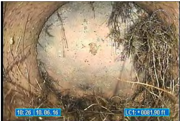
3010_6247a8b1-8071-4e8a-bd7d-95b08b3a3be1.jpg, 00:00:09, 81.90 Tap Factory Made Capped, at 10 o'clock, 6 inch dim
