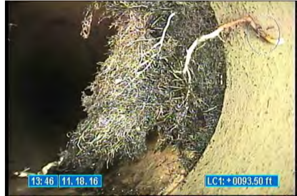
3180_1e1ea754-6f72-4874-922a-2548c4be56de.jpg, 00:00:08, 93.50 Roots Medium Joint, from 12 to 06 o'clock, within 8 inch
