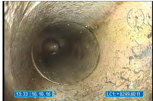
3310_f4b38433-e467-43c0-b6eb-944edd541f5b.jpg, 00:00:33, 249.60 Tap Factory Made, at 06 o'clock, 6 inch dim
