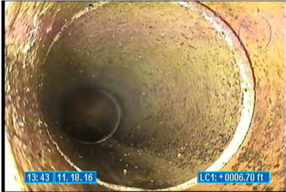
3180_d5cb02d0-fa34-4c23-96c2-7eaf189b0ee0.jpg, 00:00:01, 6.70 Tap Factory Made, at 10 o'clock, 6 inch dim
