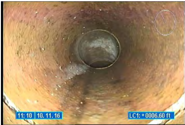
3150_34b722db-7e43-490b-a56b-06238c6aea6d.jpg, 00:00:01, 6.60 Tap Factory Made, at 10 o'clock, 6 inch dim
