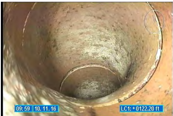
3120_fb4e99b9-5c24-439a-b064-33bf75a14cae.jpg, 00:00:22, 122.20 Tap Factory Made, at 11 o'clock, 6 inch dim
