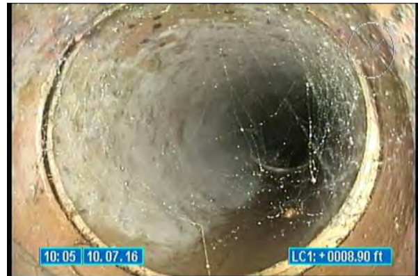
3520_832fc31b-5a54-41e5-9606-014d7f3ff1f4.jpg, 00:00:03, 8.90 Tap Factory Made, at 02 o'clock, 6 inch dim
