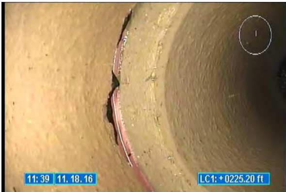
3430_2bf181ed-525c-4f25-9432-76f93918b01b.jpg, 00:00:35, 225.20 Joint Offset Medium
