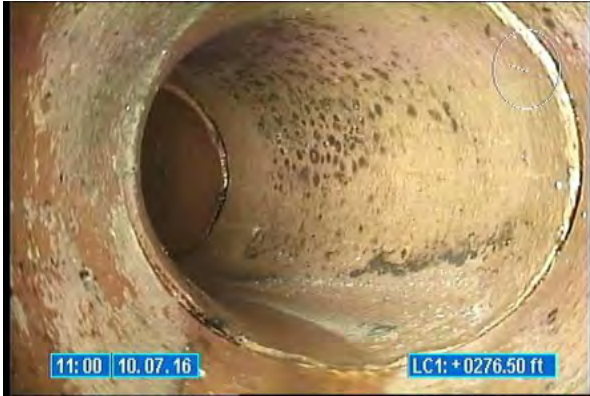
3500_5f8183c5-e27f-43a4-97d9-11db5071d392.jpg, 00:00:37, 276.50 Tap Factory Made Active, at 10 o'clock, 6 inch dim
