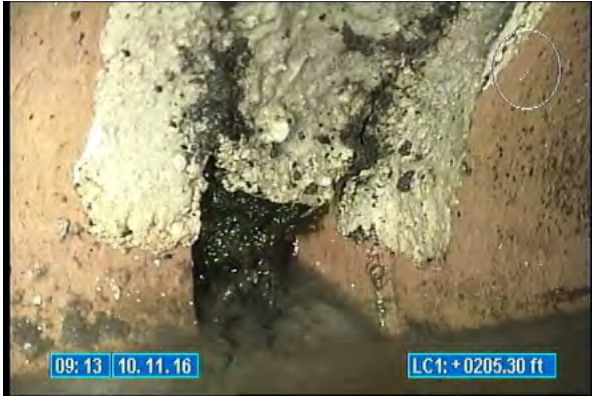
3100_ef589ddb-4e97-4021-b9f2-20ec6e2626ca.jpg, 00:00:25, 205.30 Joint Separated Medium
