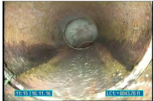
3150_36e81095-618b-4b7d-9da4-26e8bd726a25.jpg, 00:00:05, 43.70 Tap Factory Made, at 01 o'clock, 6 inch dim
