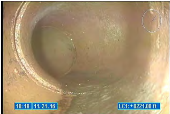
3450_c7c59913-cb0b-40dd-ab3d-70cfad8fadde.jpg, 00:00:30, 221.00 Tap Factory Made, at 02 o'clock, 6 inch dim
