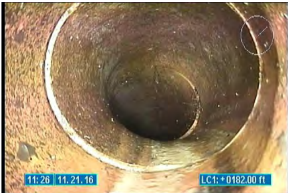
3280_21fedd0e-91c6-48f7-852a-77b8ea600c0d.jpg, 00:00:17, 182.00 Tap Factory Made, at 02 o'clock, 6 inch dim
