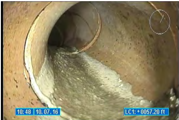
3500_cb7ec75f-5de4-4aed-ab7b-d4d7158a5fff.jpg, 00:00:08, 57.20 Tap Factory Made Active, at 02 o'clock, 6 inch dim
