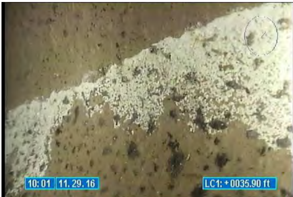
3940_54869c28-7f1d-4dbf-b46f-0a4117d66aaa.jpg, 00:00:06, 35.90 Deposits Attached Encrustation, at 02 o'clock
