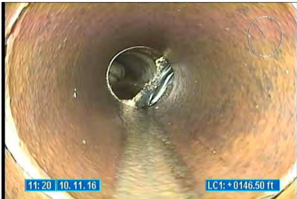
3150_ef68d233-48c2-4366-ad99-9fc3a3ab8c41.jpg, 00:00:15, 146.50 Tap Factory Made, at 10 o'clock, 6 inch dim
