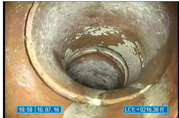
3500_496328aa-d87e-40d3-91ed-8d309d8363fa.jpg, 00:00:31, 216.30 Tap Factory Made Active, at 02 o'clock, 6 inch dim
