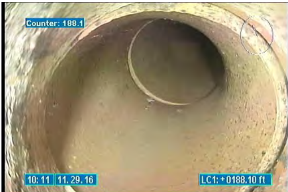
3940_05be227a-9aa7-4691-9669-ea8c4db91697.jpg, 00:00:30, 188.10 Tap Factory Made, at 10 o'clock, 6 inch dim
