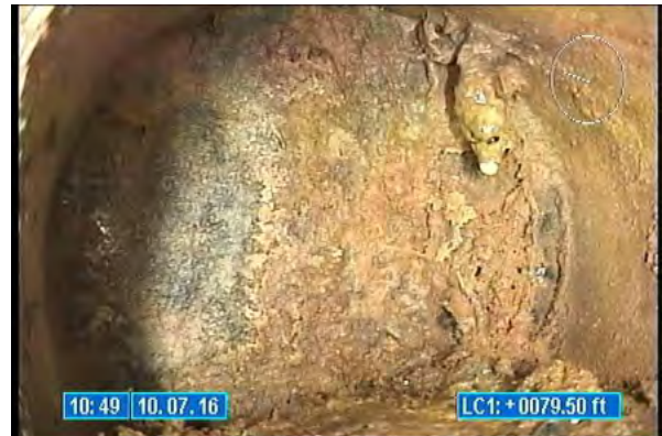
3500_f27cd354-dc0b-4295-8fd2-2886ec76f0f2.jpg, 00:00:11, 79.50 Tap Factory Made Capped, at 10 o'clock, 6 inch dim
