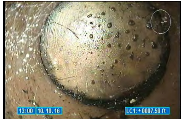
3310_0c52f952-2617-4218-8a97-349bfa18571e.jpg, 00:00:03, 7.50 Tap Factory Made Capped, at 03 o'clock, 6 inch dim
