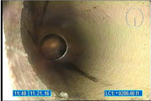
3290_a9b8b1a5-07e0-4870-932b-d384d38d5093.jpg, 00:00:26, 208.40 Tap Factory Made, at 06 o'clock, 6 inch dim
