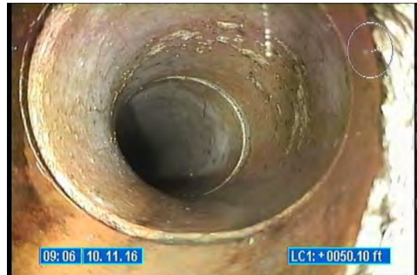
3100_88244146-1b3b-47df-af96-837b674a9958.jpg, 00:00:08, 50.10 Tap Factory Made, at 03 o'clock, 6 inch dim
