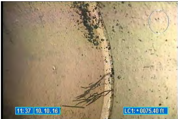
3300_95ca4457-b75e-4b6a-a0c3-2360d58d5a37.jpg, 00:00:13, 75.40 Roots Fine Joint, at 03 o'clock, within 8 inch
