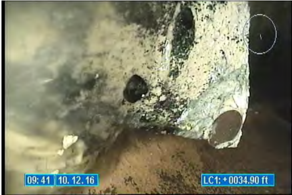
3560_ea814fa4-e7ea-4e22-91b6-fc880c59a7f5.jpg, 00:00:34, 34.90 Deposits Settled Other, at 06 o'clock
