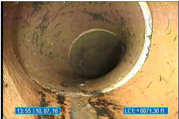
3230_8783906d-3b9c-42a3-afd8-ffcff2043b13.jpg, 00:00:08, 71.30 Tap Factory Made, at 09 o'clock, 6 inch dim
