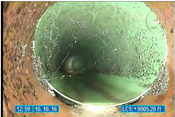
3310_40823228-b556-4d7a-b5ce-2710e7dd9235.jpg, 00:00:02, 5.20 Tap Factory Made, at 09 o'clock, 6 inch dim
