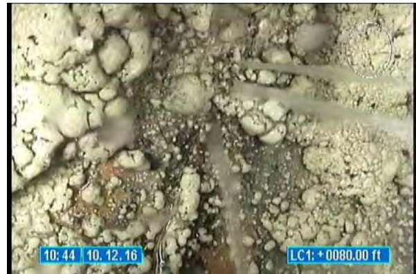
3650_790d8b17-78d1-4c9f-a5c1-4afa8ce40de6.jpg, 00:00:11, 80.00 Fracture Circumferential, from 12 to 12 o'clock
