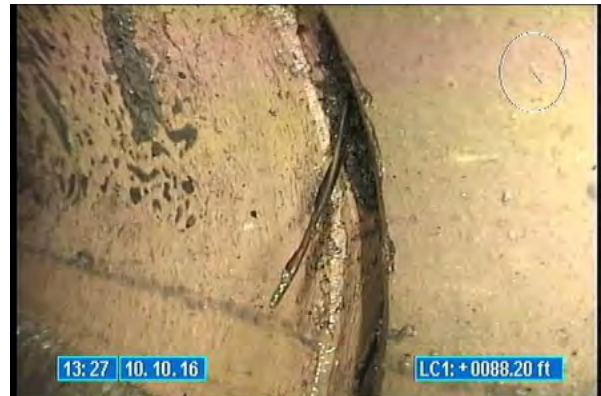
3310_cd67154b-d8c0-4490-b304-b108d8d528cd.jpg, 00:00:18, 88.20 Roots Fine Joint, at 04 o'clock, within 8 inch
