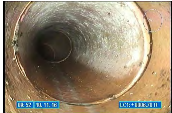
3120_a82aec60-b12a-495e-be0b-0764d502d342.jpg, 00:00:06, 6.70 Tap Factory Made, at 10 o'clock, 6 inch dim
