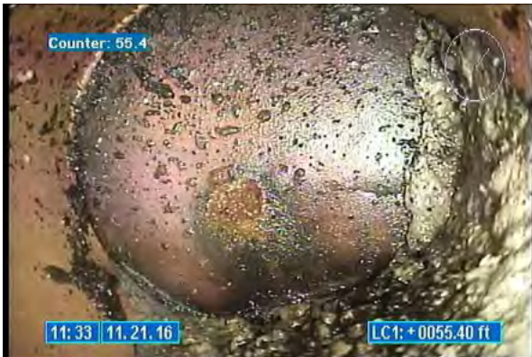
3290_962e0a4f-bfdb-46f2-99ff-4c3c9a8a600f.jpg, 00:00:09, 55.40 Tap Factory Made Capped, at 02 o'clock, 6 inch dim
