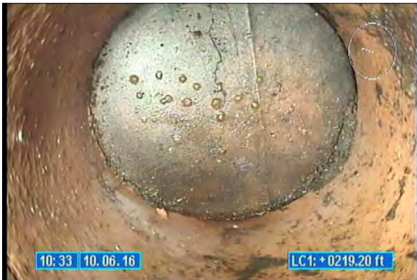
3010_262b5cf4-236c-4fd3-bebf-8b4da6551b76.jpg, 00:00:26, 219.20 Tap Factory Made Capped, at 10 o'clock, 6 inch dim
