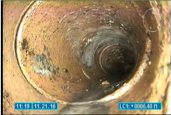
3280_df35267c-2048-43bb-a086-fab28dfb3300.jpg, 00:00:01, 6.40 Tap Factory Made, at 02 o'clock, 6 inch dim
