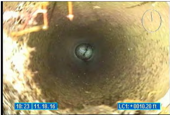
3350_4f80a37f-1843-485e-82ea-6b0765d81f4f.jpg, 00:00:05, 10.20 Tap Factory Made Capped, at 11 o'clock, 6 inch dim
